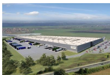
Goodman Wrocław South Logistics Centre (Amazon) 123.500 mkw.
